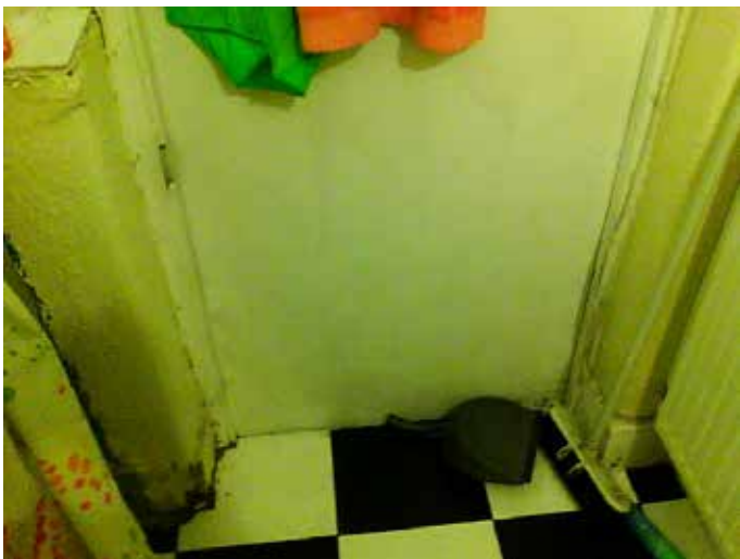
Heat-loss around external door to balcony. Improved draught-stripping here could significantly reduce this.
