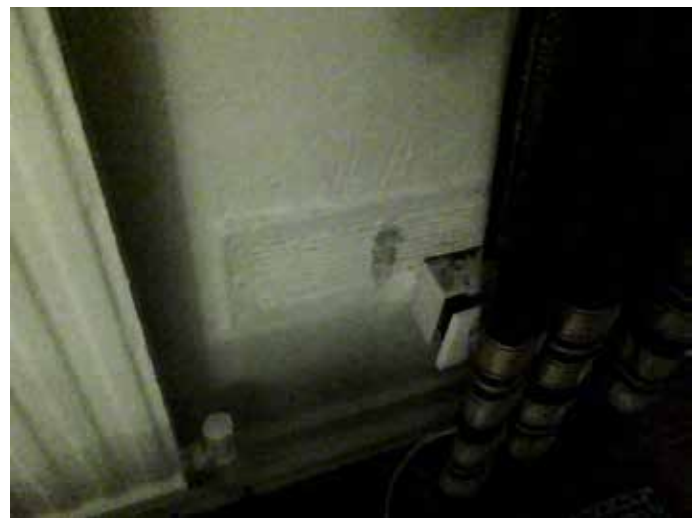
Lots of draughts and leaks are caused by poorly-sealed building services - such as around waste pipes from bathrooms. It's a relatively simple job to just seal these better.
