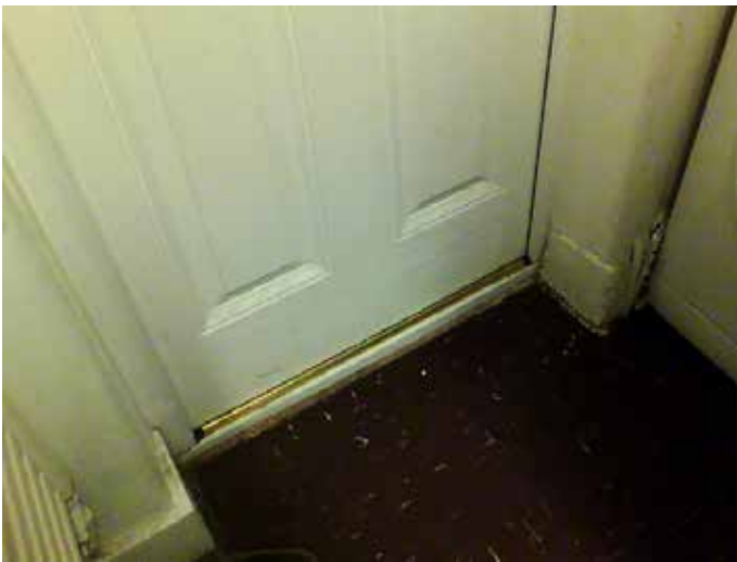
Heat-loss at flat entrance door threshold - some draught-proofing, but could be improved.
